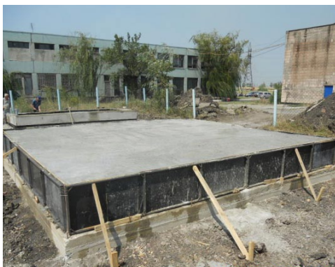
Site preparation and foundations
