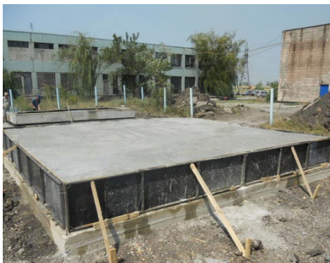
Site preparation and foundations
